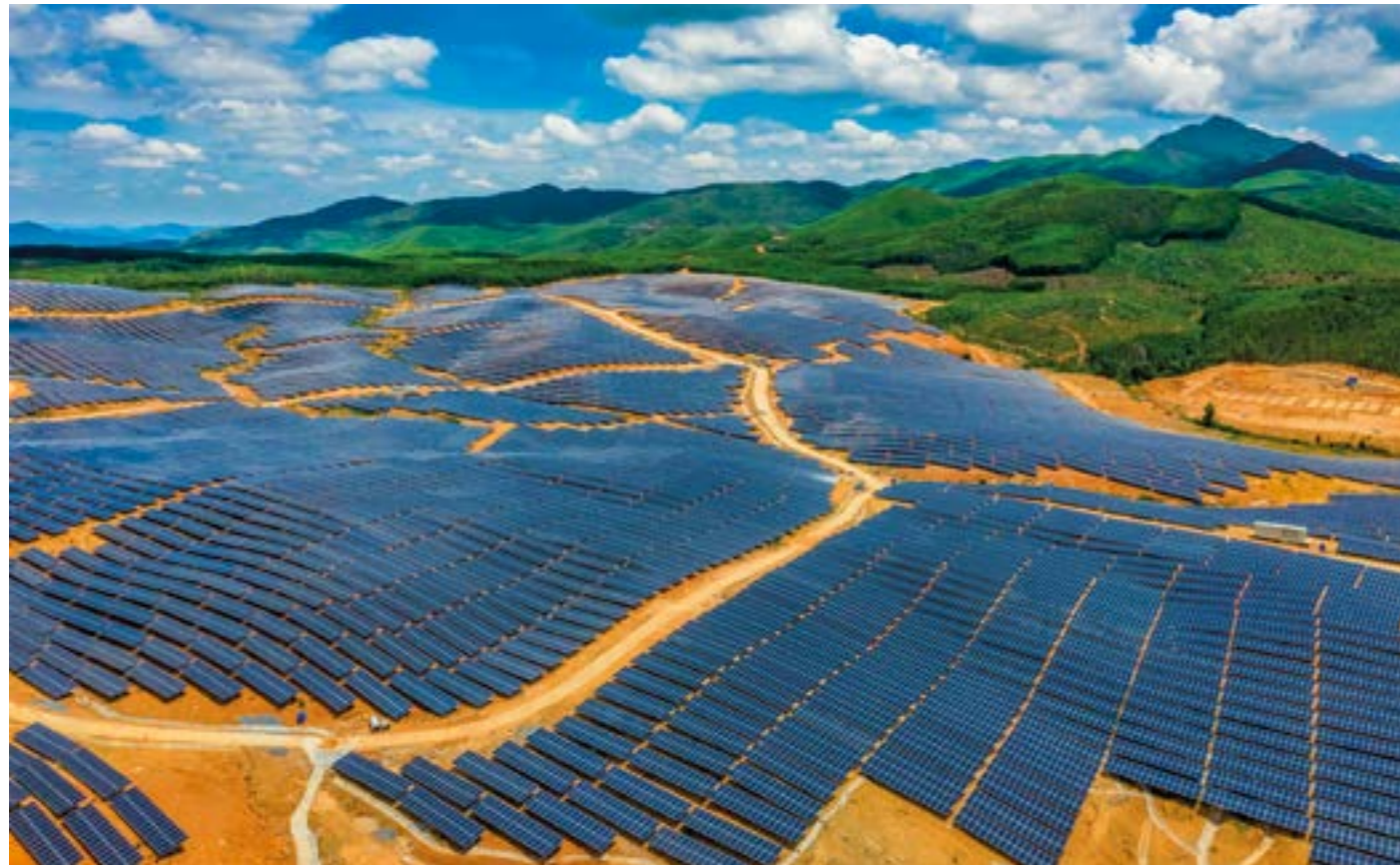
An aerial view of photovoltaic panels at Xuan Tho, Song Cau, Phu Yen, Vietnam. Source: Shutterstock
